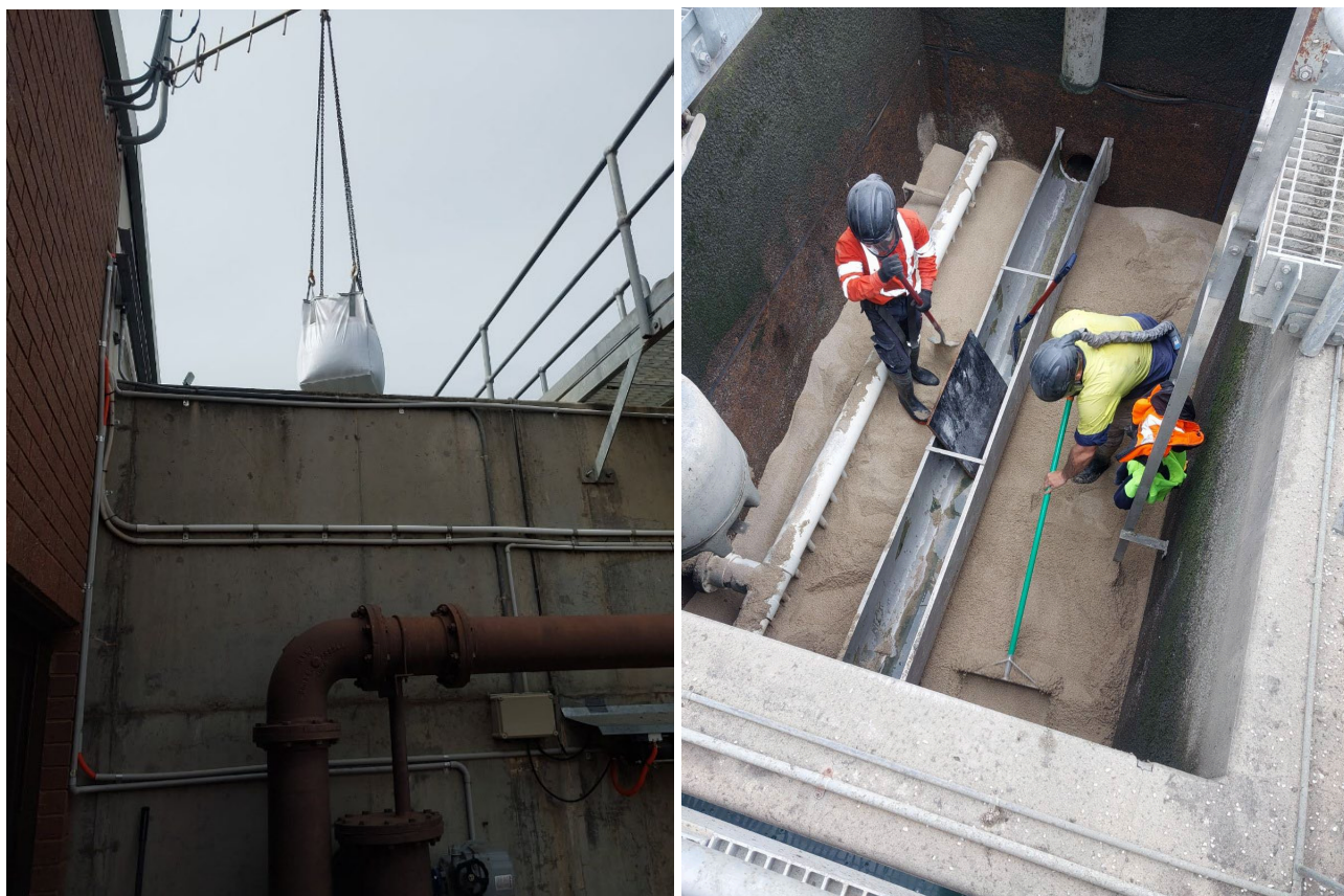
Filter media replacement at the water treatment plant
