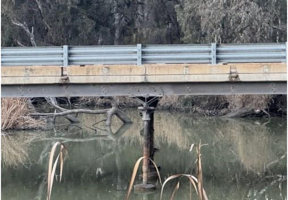
Figure 8: Rolled wrought iron joists and angle plates used to brace the transverse beam.
