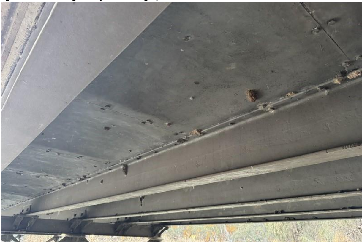
Figure 9: Rolled wrought iron joists shown below the deck with mild steel plates bolted to the beam flanges.
