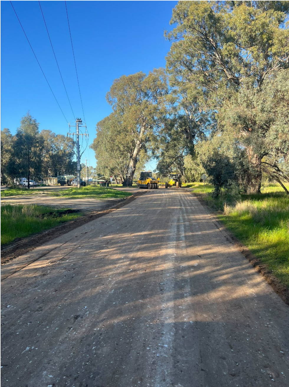
Sandy Point maintenance grading access roads
