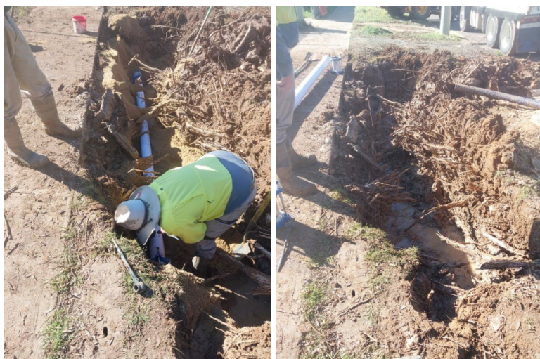
Water main repairs in Cadell Street
