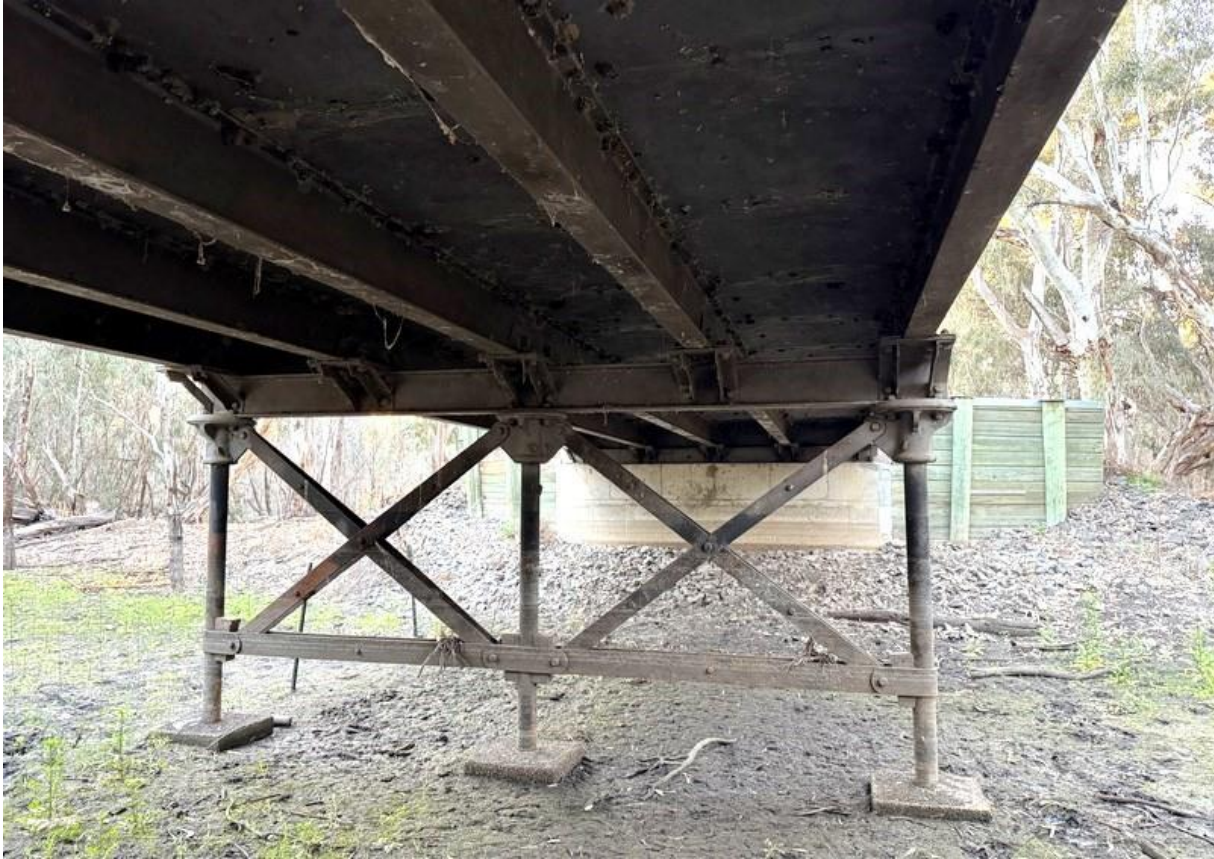
Figure 12: Central pier under the Oxley bridge, showing rolled wrought iron bracing bars and clips. Note, as well, the rolled wrought iron joists and replaced metal sheeting that has been bolted to the flanges.
