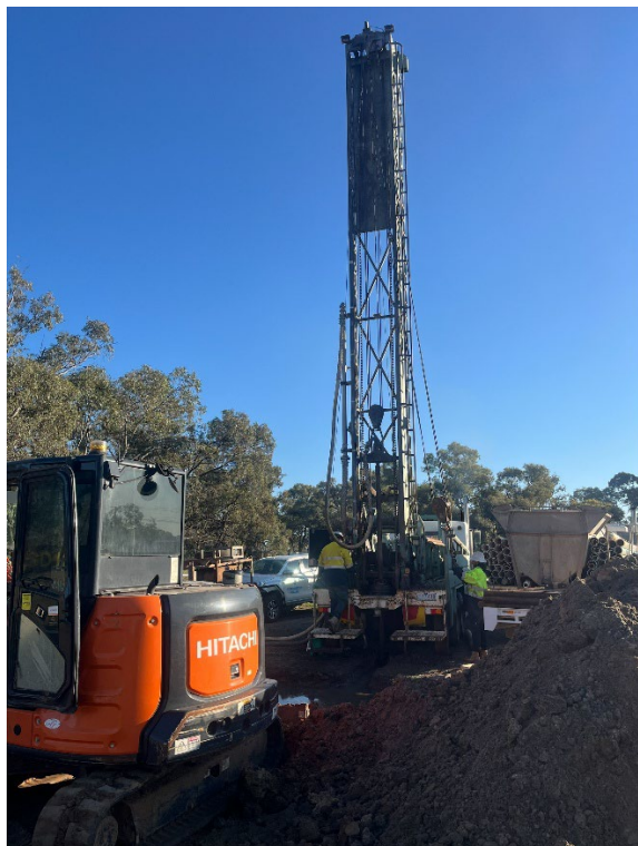
Drilling secondary water supply for water quality testing
