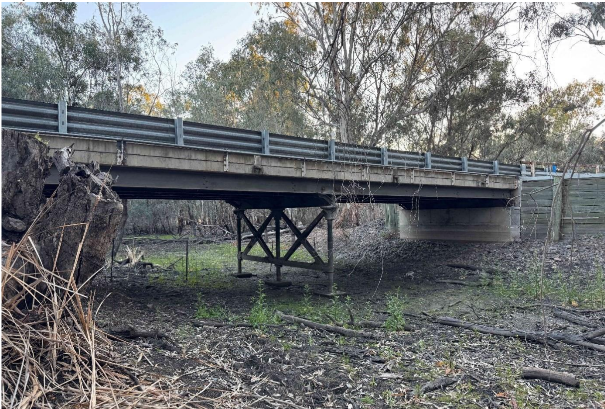
Figure 11: Overview of Oxley Bridge No.2 showing rolled wrought iron beams, deck and piers in its setting on Cumbung Creek.
