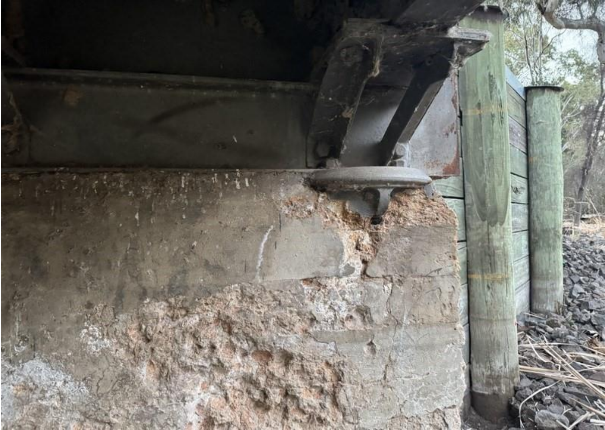
Figure 10: Lime mortar concrete headwall on the eastern side of the embankment showing an embedded cast iron pile cap.
