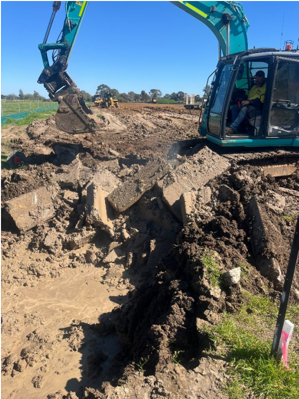
Concrete removal from subgrade at HVRA
