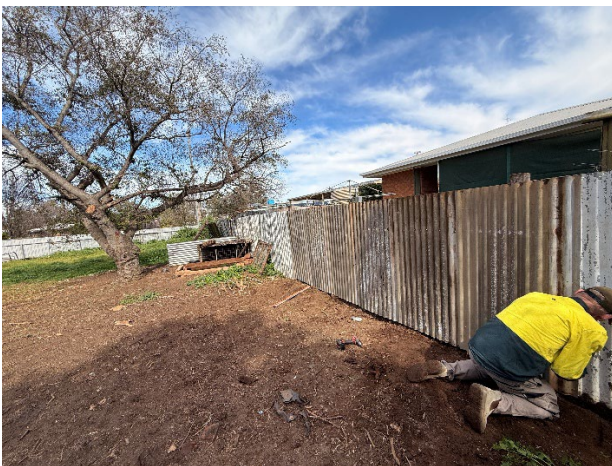
Fence repairs after sewer repairs
