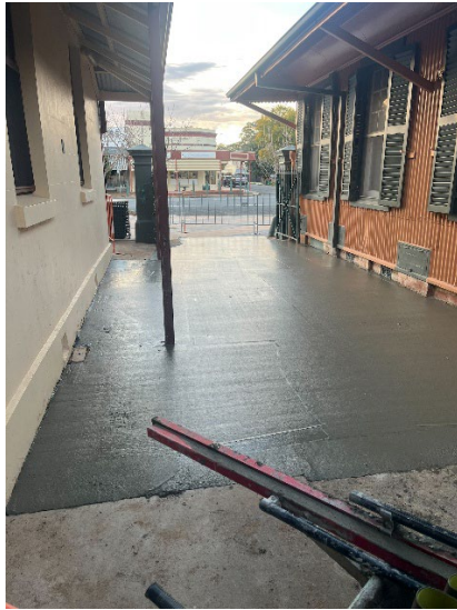
Concrete replacement after NBN works
